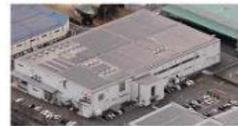
Japan Toyohama Manufacturing Site
