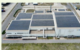
Tianjin packaging factory
